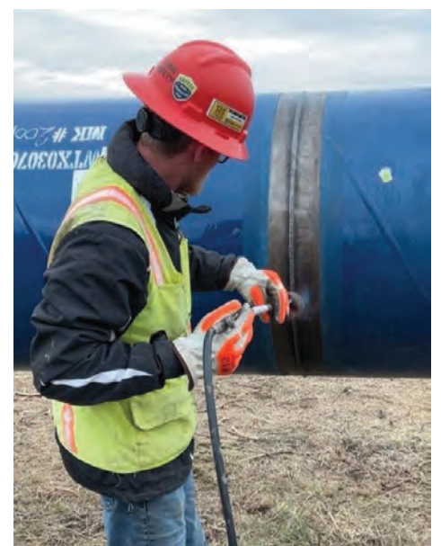
Seg E – Preparing Pipe for Epoxy
