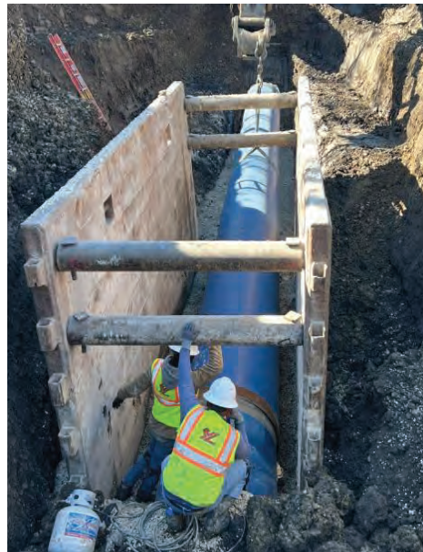
Seg D – Pipe Placement
