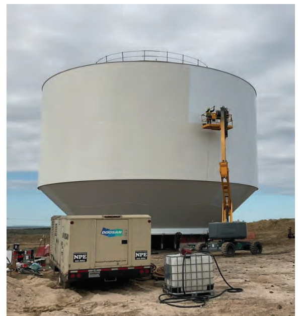
EST – Rolling on Final Coat of Paint
