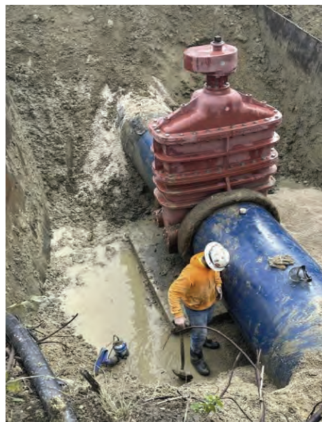
Seg B – Cleaning Gate Valve by SH-130
