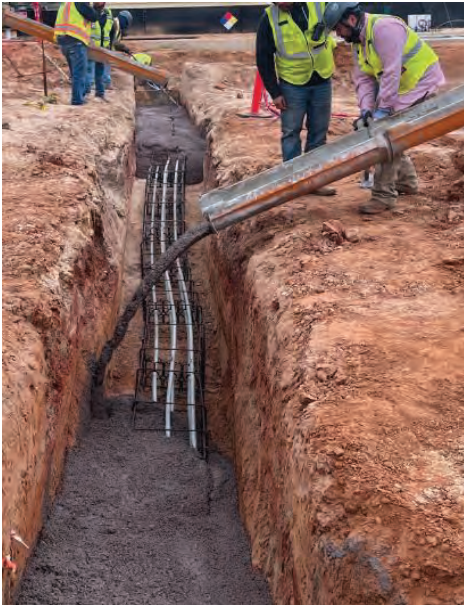
WTP – Duct Bank K-K Concrete Placement
