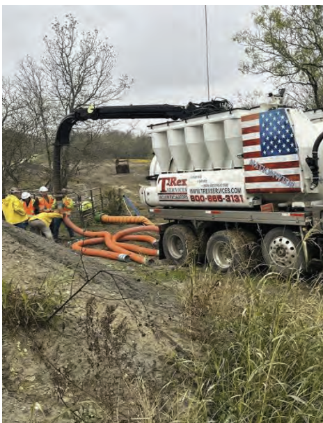
Seg B – Vacuuming Debris from SH-130 Tunnel
