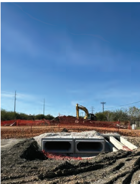
BPS – Installing Base Material for Access Road
