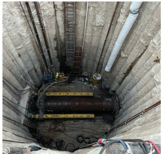
Seg D – Micro tunnel Shaft
