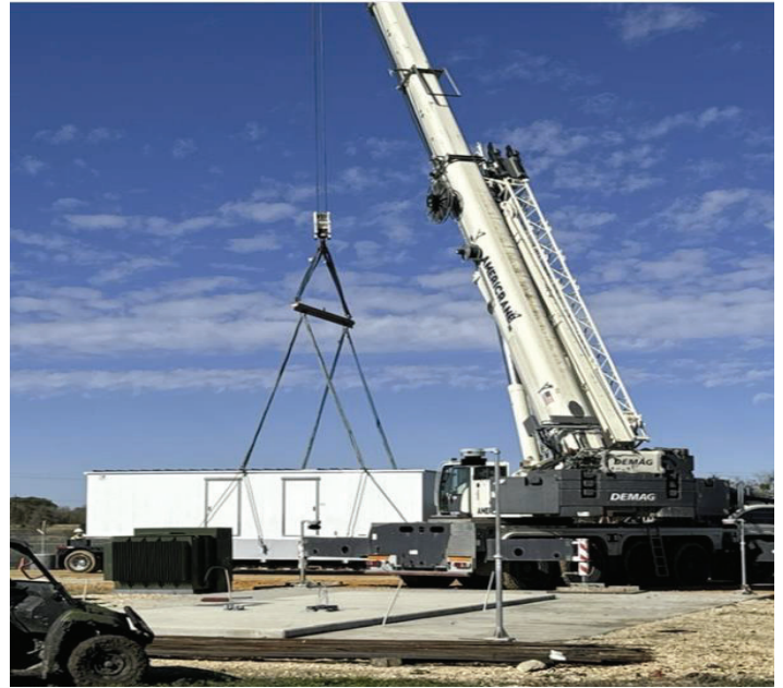
BPS – Offloading BPS Generator
