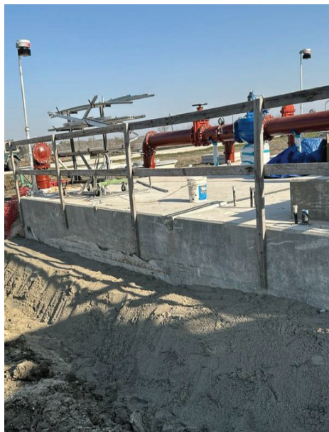
BPS – Flow Fill Placement Around Pump Station
