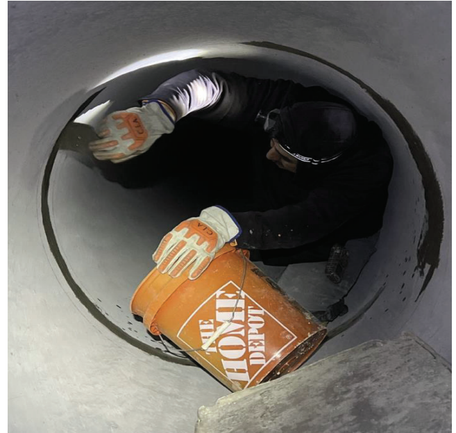
Seg E – Grouting Cracks in the Concrete Liner
