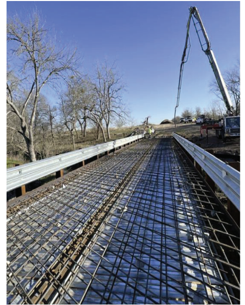
Seg D – Rebar Mats Placed and Ready for Concrete
