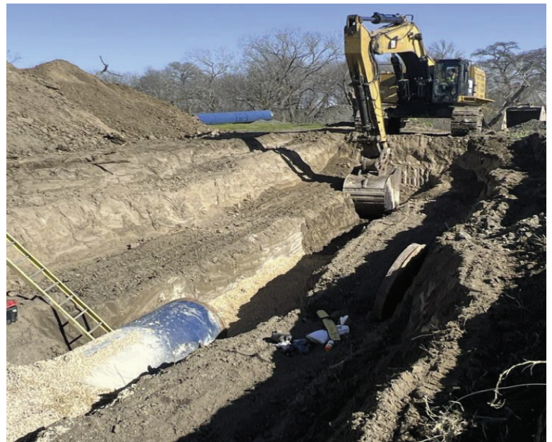
Seg D – Trench Preparation
