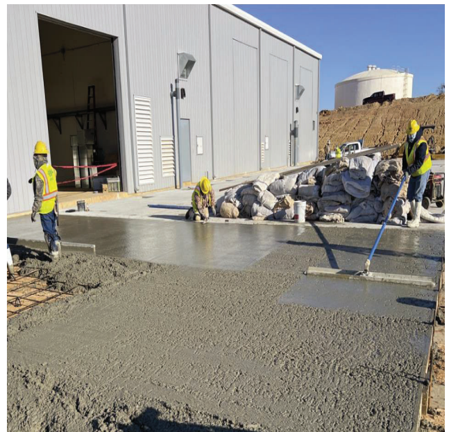
WTP Drive 2 Concrete Placement
