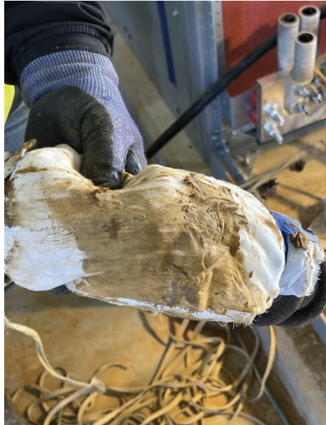
WTP – Cleaning Duct Bank Conduits
