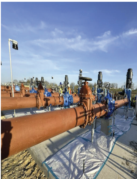
BPS – BPS – Coating Prep Work
