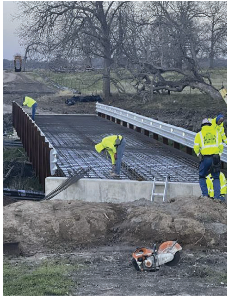
Seg D – Tying Rebar for Concrete Deck on Morrison Creek Bridge
