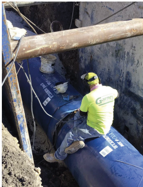
Seg E – Welding Clips into Place
