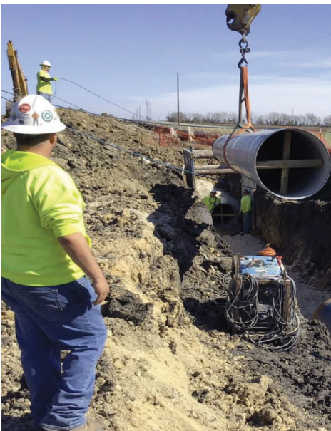
Seg E – Setting Pipe into Place
