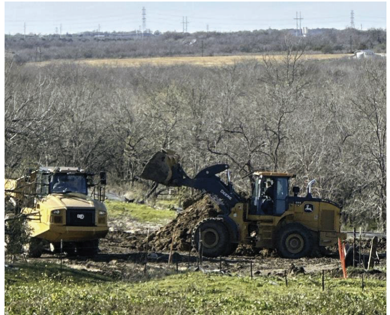
Segment B – Removing Spoils Near Boggy Creek
