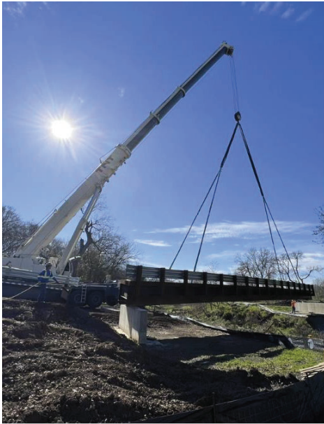
Seg D – Crane Setting Preassembled Sections of Morrison Creek Bridge
