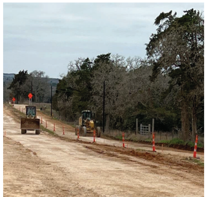
WTP – Grading Sides of Wolf Run Road
