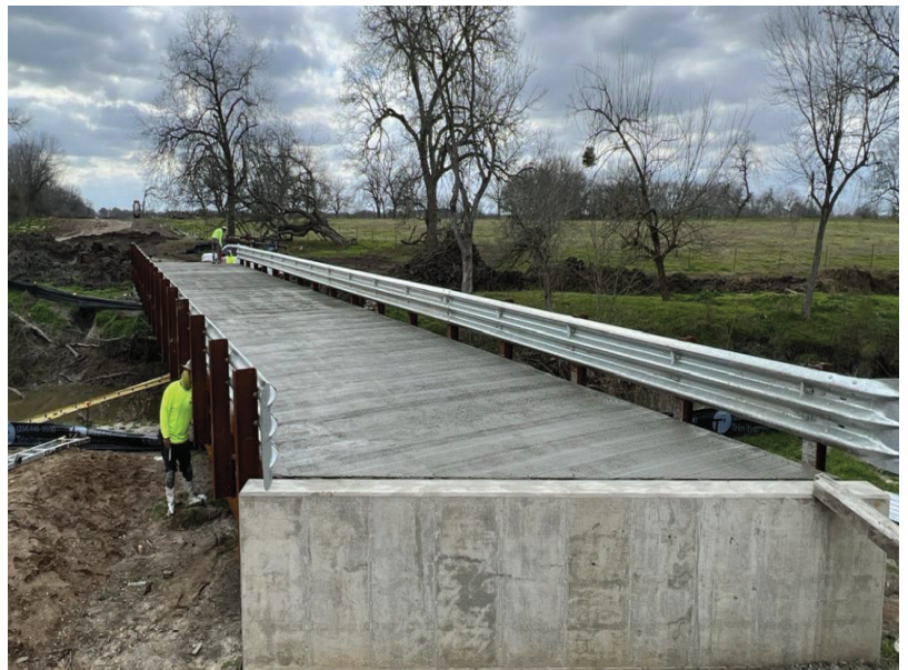
Seg D – Morrison Creek Bridge Cleanup
