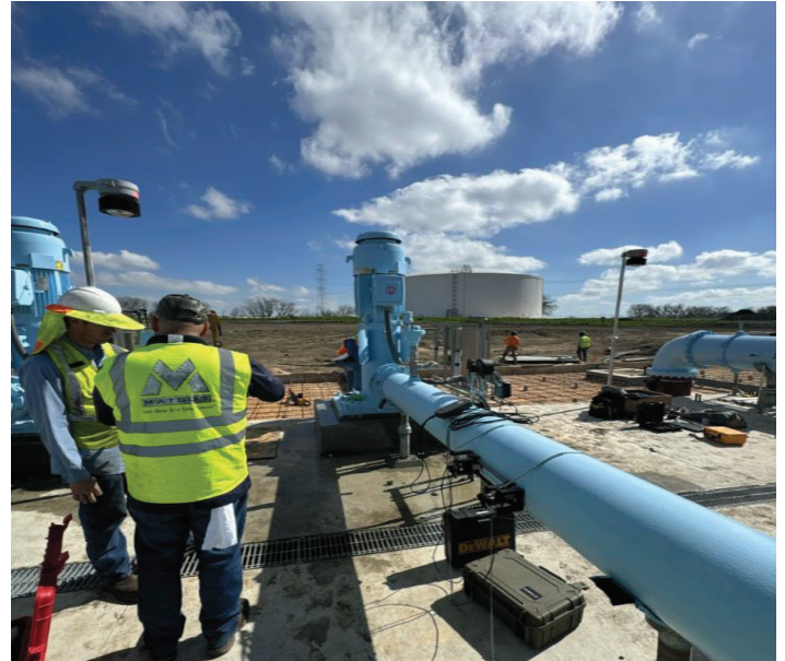
BPS – Segment C Testing
