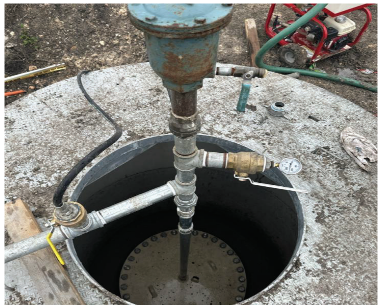
Segment B – Hydrostatic Testing Line B1
