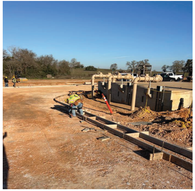
WTP - Drive 2 Setting Ribbon Curb Forms
