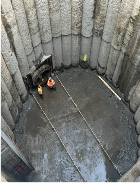
Seg D – Prepping Shaft to Push Carrier Pipe
