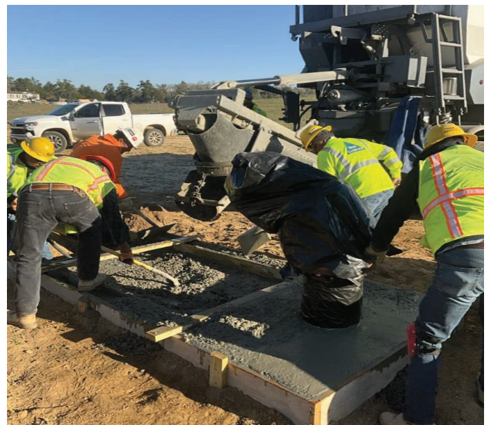
Seg A - Garney Places Concrete for Splash Pads
