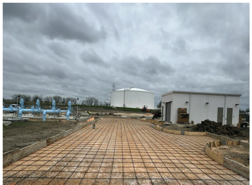
BPS – Rebar for Road Paving between PS Slab & Electrical Building
